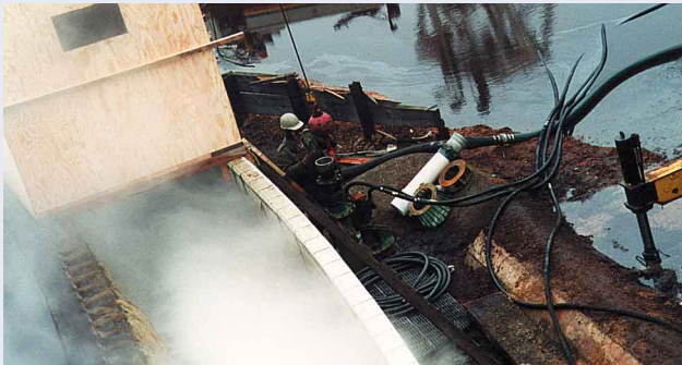
Photos above and below: SIMPSON TACOMA KRAFT PAPER MILL - Pumping a three million gallon clarifier
