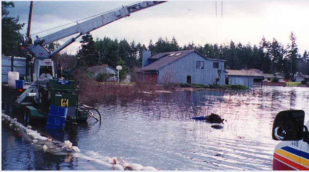
PIERCE COUNTY SURFACE WATER MANAGEMENT (SWM)- By-pass pumping
