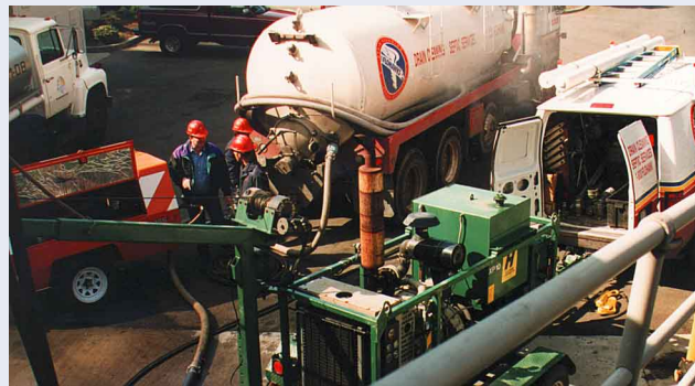
SOUTHWEST SUBURBAN SEWER DISTRICT - Digester cleaning in Normandy Park
